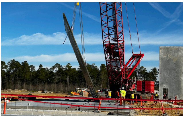
Concrete slab weighing 4,000 lbs lifted by heavy duty crane
