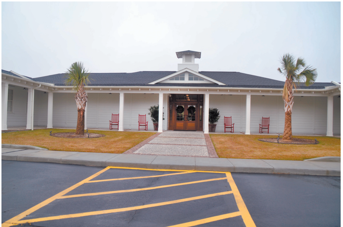
The entire airport terminal building got a face-lift, inside and out, completed in summer 2019. In addition to the conference room above, there is a small kitchen, a smaller lounge, a pilot's lounge and a large restroom with a shower.
