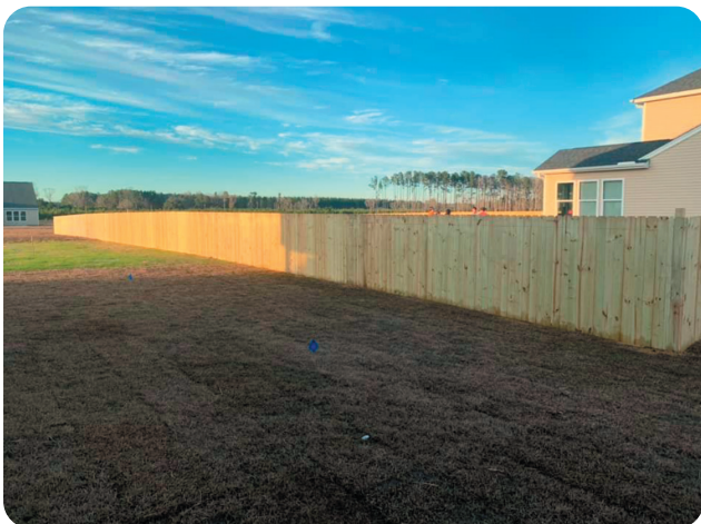
400+ ft of privacy fencing
