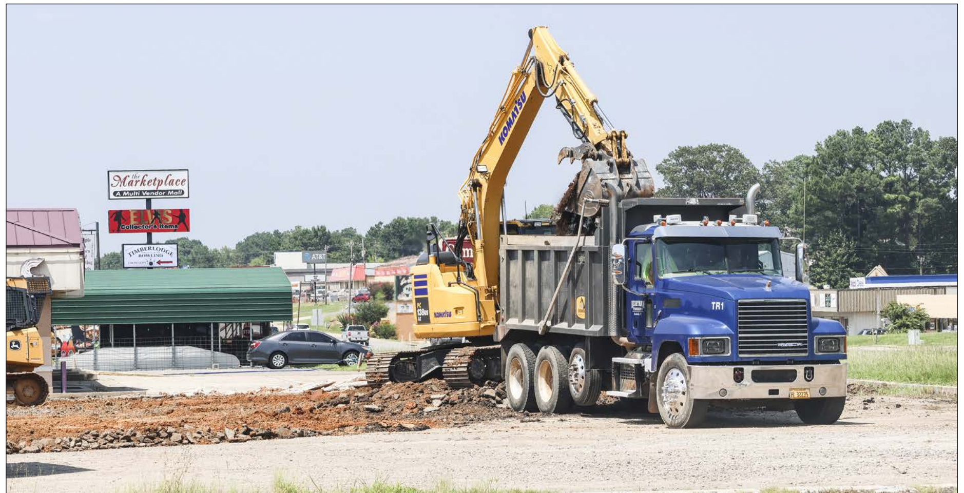
Construction crews beginning work on the site of the future Arby's.
