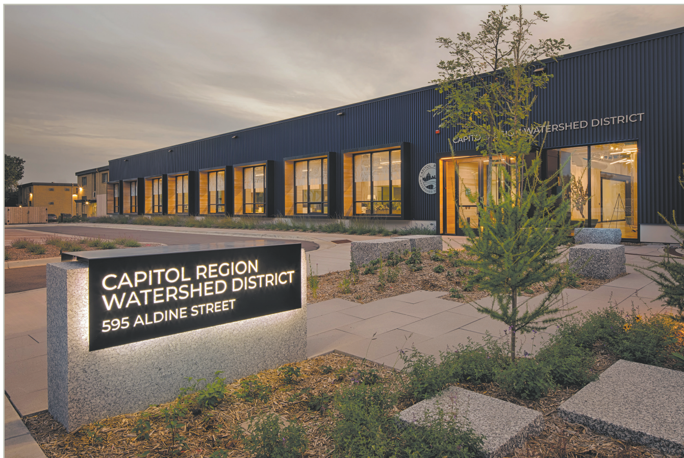
The Capitol Region Watershed District opened its office in the Midway in 2019 at the former MacQueen Equipment building.
