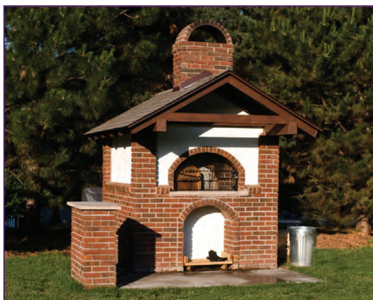
The handsome community oven at Hamline United Methodist Church takes 10-12 hours to rise to its baking temperature of 900+ degrees. Made of high-temperature concrete, clay bricks and wool insulation, the traditional design keeps the high heat on the inside. On the outside, it's barely even warm to the touch.
