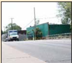
Rice St. Bridge project underway
