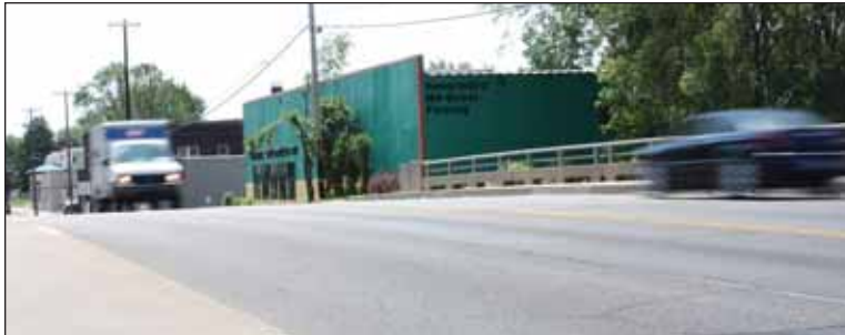
The bridge project start date hasn't been set but will be announced soon. It will mean several weeks of detours and a truncated Rice Street Parade. The parade typically crosses the bridge and ends at Arlington Senior High School. This year it will end at Ivy. (Photo by Liberty Willms)
