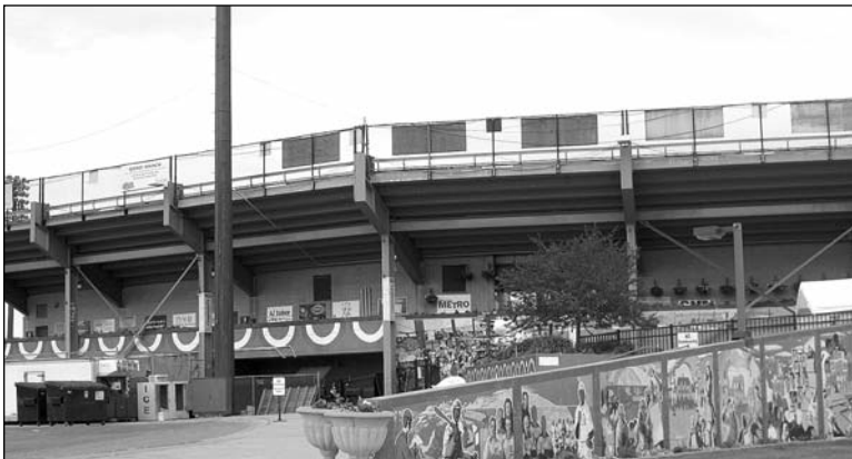
An agreement has been reached with United Properties to redevelop the Midway Stadium site. The Port and United Properties will co-own and operate the property, which is expected to become a mixed commercial and industrial site. Demolition and site cleanup will start after the last ballgames are played.
