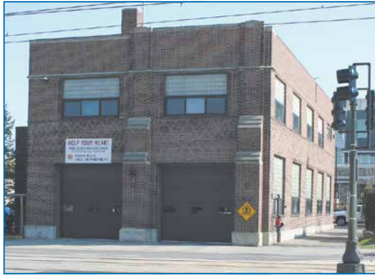
The fire station at 2179 University Ave. (Staff photo)
