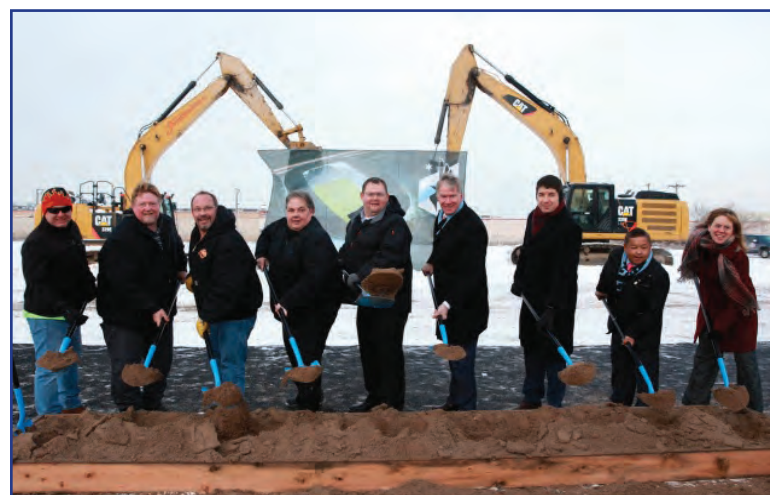
About 200 people showed up to break ground for the new soccer stadium on Dec. 12. Dozens took turns wielding shovels in a raised garden bed since the ground was frozen. (Photo submitted)
