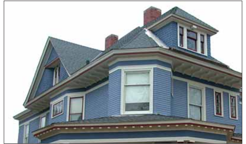
Brad Nilles, of Nilles Builders, Inc., which has been in business for 30 years, says people in the Como Park, North End, and Midway areas are doing infrastructure improvements such as rain gutters, siding, and roofing.
