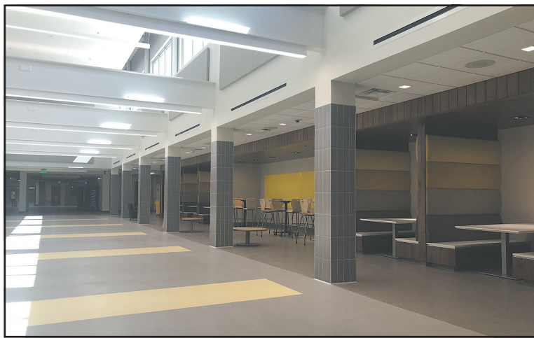
Summer construction at Como Park High School included the completion of the Como Commons.
