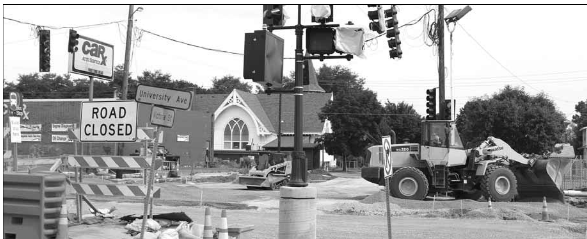
Concrete barricades, dug-up streets and blocked sidewalks are hurting businesses and angering residents. One of the biggest complaints is how north-south intersections are being rebuilt and how traffic is rerouted. (Photo by Stefanie Berres)
