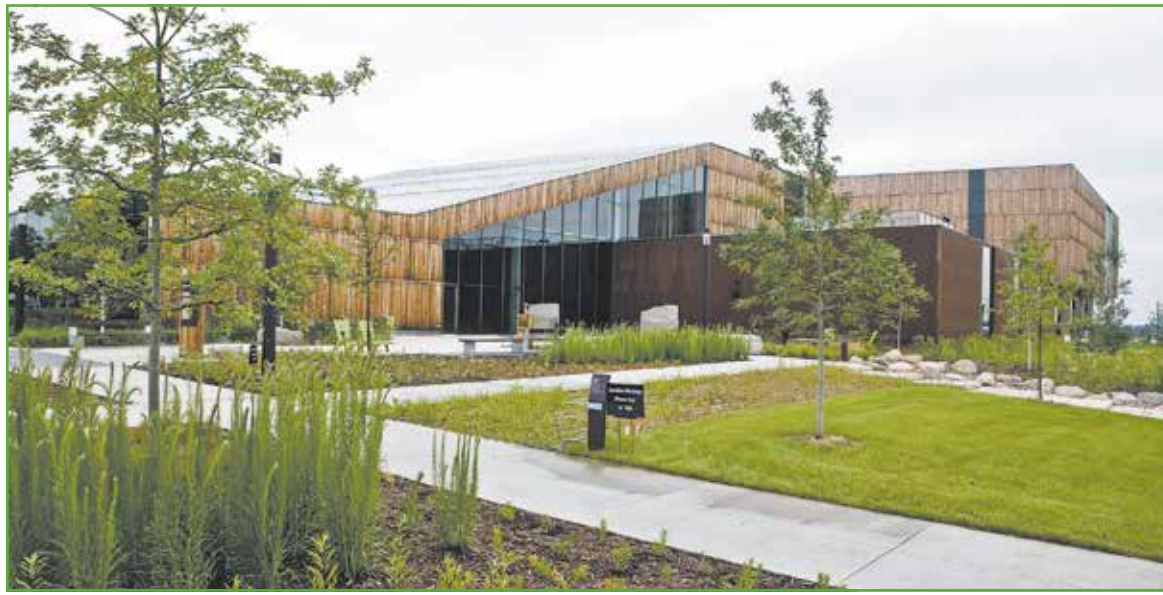
The new Bell Museum features 60% more public space than its previous location. Located at the intersection of Larpenteur and Cleveland avenues, the museum proudly features local, sustainably sourced materials such as white pine from Cass Lake, granite from south central Minnesota, steel from the Iron Range, native plants from across the state, and bird-safe glass manufactured in Owatonna. Total cost for the new museum is $79 million, and came from a combination of state funding, the University of Minnesota, and private donations. (Photo by Margie O'Loughlin)
