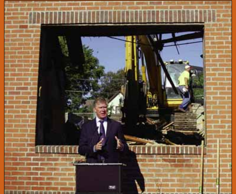
Saint Paul Mayor Chris Coleman, Councilmember Lee Helgen, local officials and community leaders celebrated last week as a long vacant building at 855 Rice collapsed into a pile of rubble. Standing empty for 22 years, the adjacent structure at 857 Rice Street will be renovated to house Libby Law Office and their tenant, Sparc, a community development organization.
