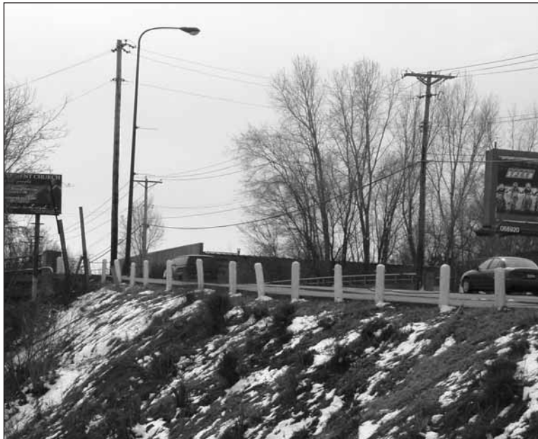
Without approval of plans soon the Rice Street Bridge reconstruction project could be pushed back until 2009.
