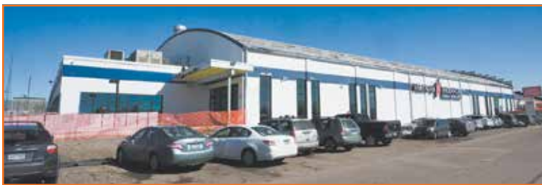
Vertical Endeavors Twin Cities Bouldering as seen from the front. An extensive parking lot is to the left. Easy access from the LRT is just two blocks to the north. (Photo by Margie O'Loughlin)
