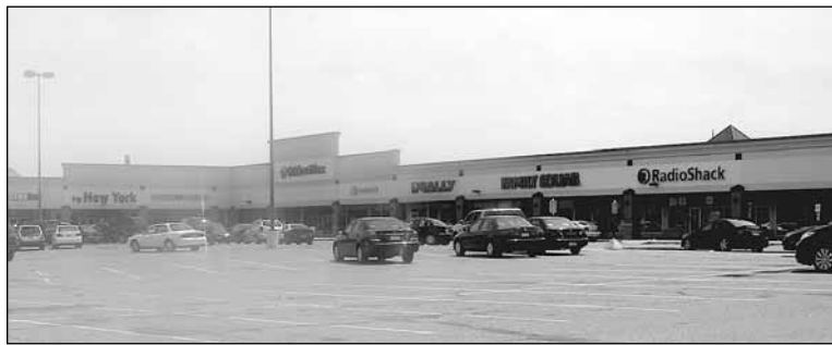
With multiple agencies involved, in addition to the owner and the city, a longer-term plan to develop the Midway Center site seems to be moving along, but at a snail's pace.
