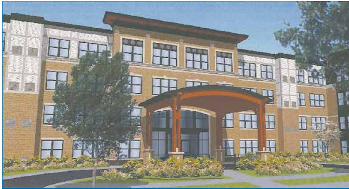
The concept drawing for the Legends of Berry front entrance at 777 and 778 Berry St. The proposed developments each have a covered front walkway with a zero setback, driving the need for a variance from the regulation requiring a 10 foot setback. (Illustration provided)
