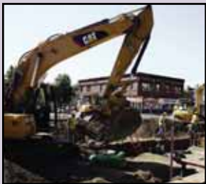
Central Corridor work starts again
