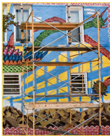
With scaffolding in place, Yuya Negishi and assistants are working on changes to the Midway Mural Project at 689 Snelling Ave. As of the last week in September, the rising sun has been removed, and the rays of the sun are being replaced with a grid pattern that will transition to blue skies overhead. (Photo by Margie O'Loughlin)
