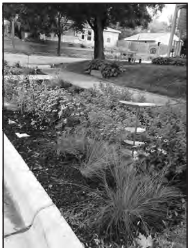
Rain gardens slow stormwater runoff while adding beauty to our streets.
