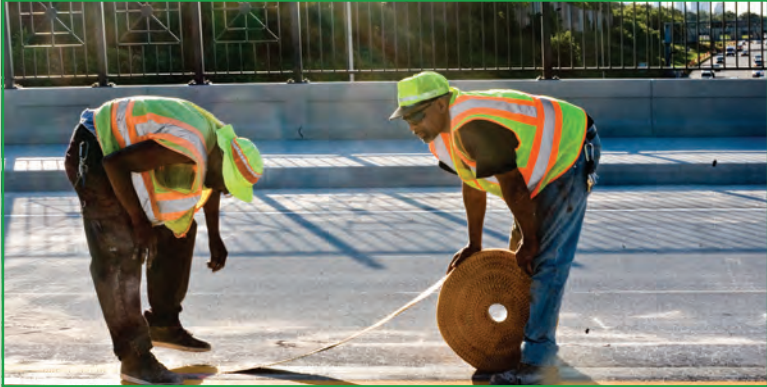
Crews worked up until the last minute marking and taping lane dividers. The new bridge has 10' wide sidewalks, 6' wide bike lanes and 6' wide buffers in both directions and 12' wide lanes for automobiles.
