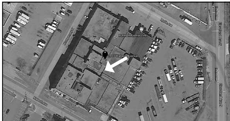
You can see from this satellite image the complexity of the building by all the site line changes in the roof. The oldest part of the structure dates from 1886. It was added onto in 1911, 1928 and 1947, so it has different floor levels and roof heights. Sections range from one to three stories in height. (Web image)
