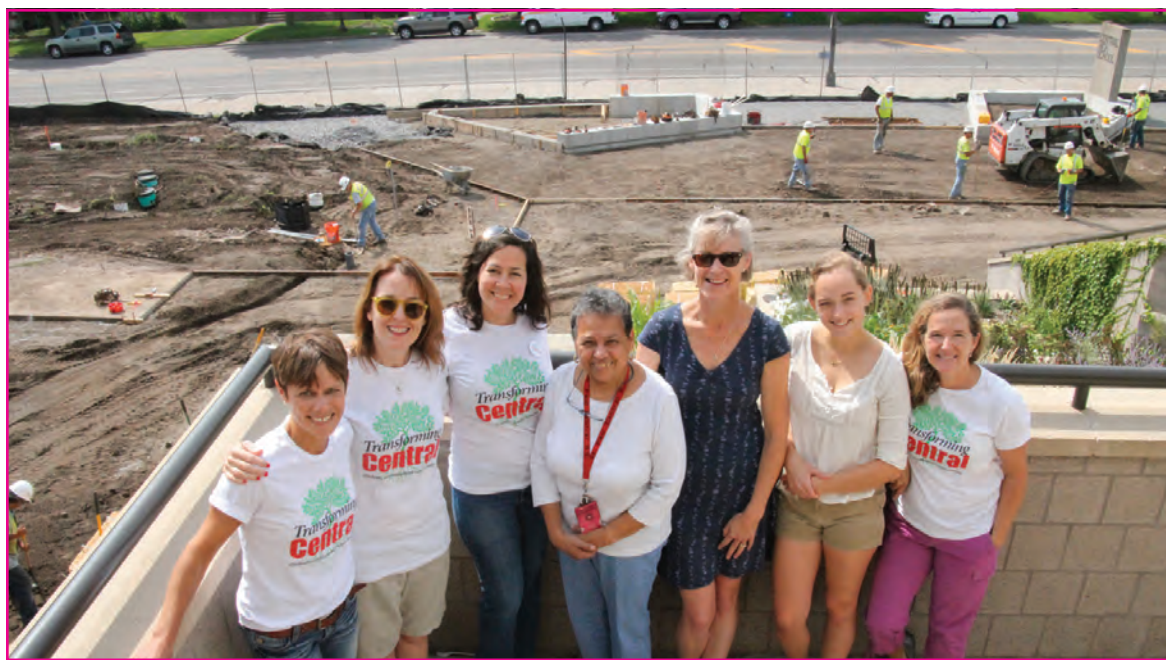
Members of the Transforming Central Committee are excited to see five years of work coming to fruition. The changes to the stormwater system and front plaza were sparked by students, staff, and parents. The project completion kicks off the sesquicentennial celebration of the school. Left to right: Ann Hobbie, Lisa Heyman, Maggie O’Reilly, Principal Mary Mackbee, Julie Marckel, Olive Murdoch Meyer and Nina Tuttle. (Photo by Tesha M. Christensen)
