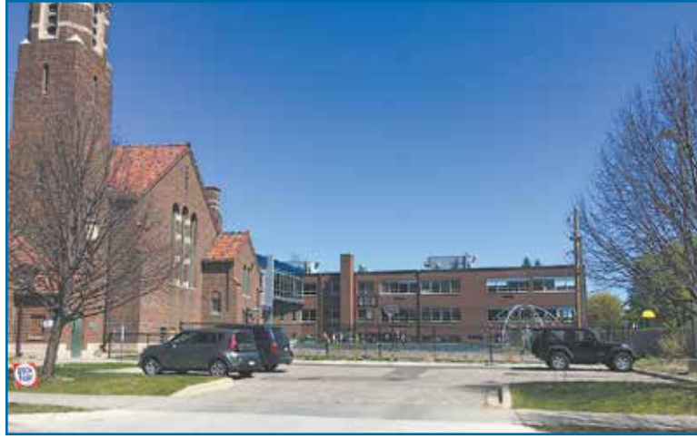
The Twin Cities German Immersion School has outgrown its current building at 1031 Como Ave. and plans to expand on its existing site. The expansion most likely will require extensive renovation or replacement of the old Saint Andrew's church building. (Photo by Tesha M. Christensen)
