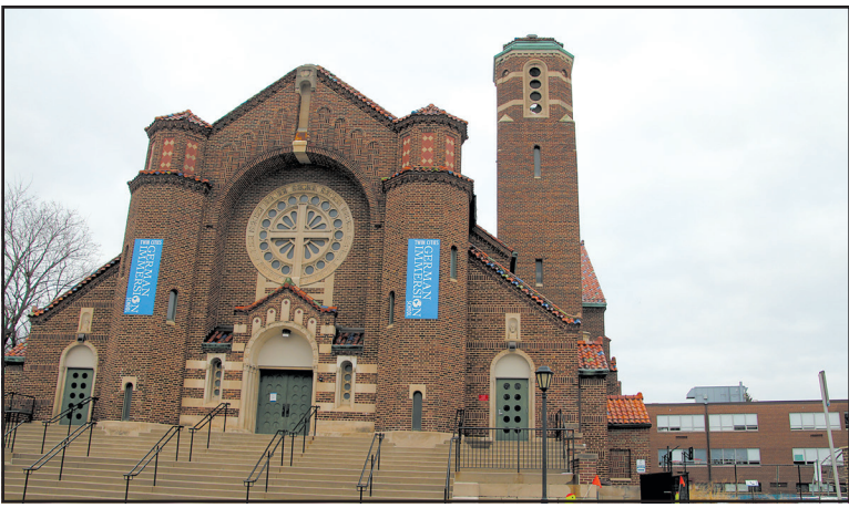
St. Andrew's was designed by St. Paul's first architect, Charles A. Hausler. (Photo by Tessa M. Christensen)
