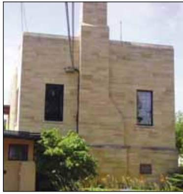
The Hamline Park Playground building will be rezoned to accommodate the pending move of Mosaic on a Stick there.
