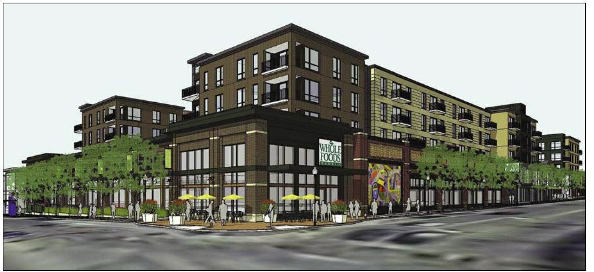
The Vintage on Selby, Ryan Companies' mixed use development at Selby and Snelling, will bring 208 dwelling units, a Whole Foods store and a new bank to the area. The project won St. Paul Planning Commission approval in December.
