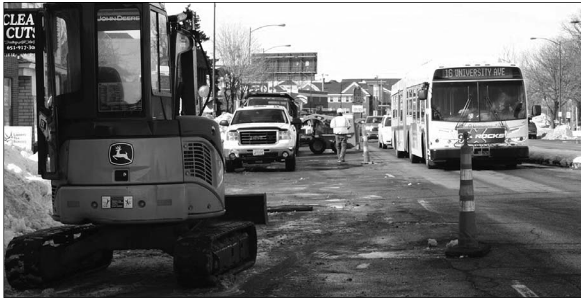
Over the past several weeks many bus stops have been removed or relocated to accommodate Central Corridor light rail construction. (Photo by Stefanie Berres)
