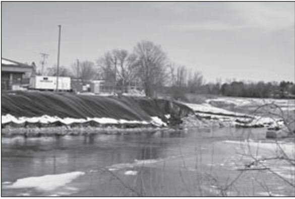
The shoreline stabilization began early spring at the Manawa dam site to ensure the northside of the river’s shoreline stops eroding into the river.
