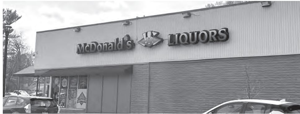
McDonald's Liquor used the grant to pay for an awning (above), while Nokomis Tattoo (at right) paid for a mural and windows. (Photos by Sarah Friedman)
