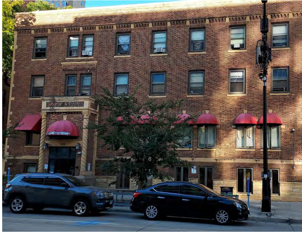
On Sept. 19, 2024, the city council approved redistributing some funds from 15 departments to pay for repairs at the Agate Board and Lodge Housing and Shelter Facility (510 South 8th St.), where Agate has a 42-bed shelter program and 95-bed board and lodge program. (Photo by Cam Gordon)
