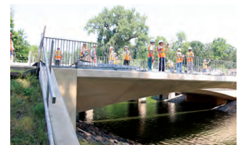
The Green Line Extension crosses the Kenilworth Channel on a bridge and then dips underground to travel under Cedar Lake Parkway. (Photo by Tesha M. Christensen)
