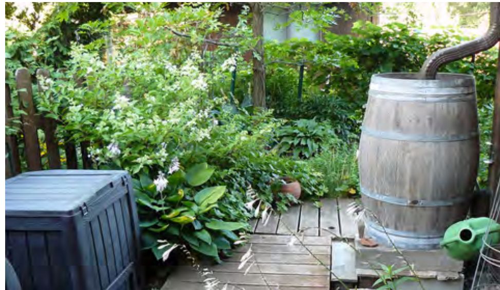
A rain barrel collects roof runoff so you can save the rainwater for later use. Reroute downspouts away from pavement and onto grass, a rain barrel or a rain garden. (Photo courtesy of the University of Minnesota Extension)
