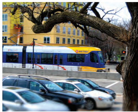
The past winter's cold snap and thaw damaged nine areas of rail, including eight areas along the Green Line. They will be fixed April 19-21.
