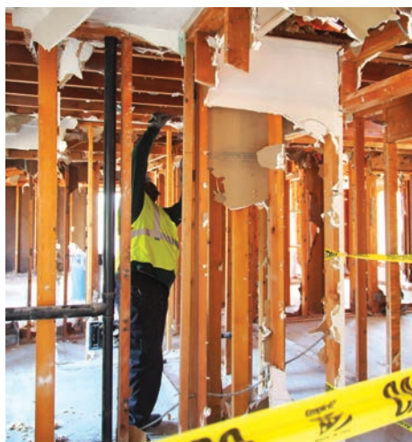
Better Futures employee de-nailing lumber in a 1960s rambler. Once the roof comes off the house, the lumber that's holding it up can be fully removed and sold at the ReUse Warehouse. (Photo by Margo Ashmore)
