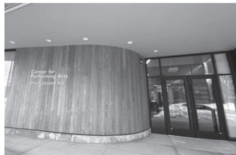
A new sidewalk porch off 38th connects the old with the new and welcomes the public in. (Photo by Tesha M. Christensen)
