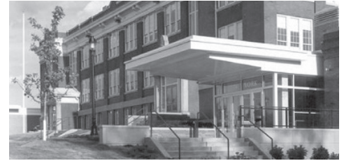
The Johnson building
