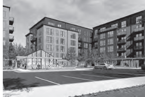
The two buildings at Wirth on the Woods in the Bryn Mawr neighborhood at 2800 Wayzata Boulevard will be named The Theodore and The Eloise. A groundbreaking was held on July 14, 2022.
