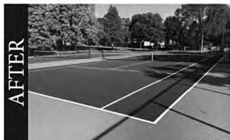
Tennis court improvements at Kenny Park.
