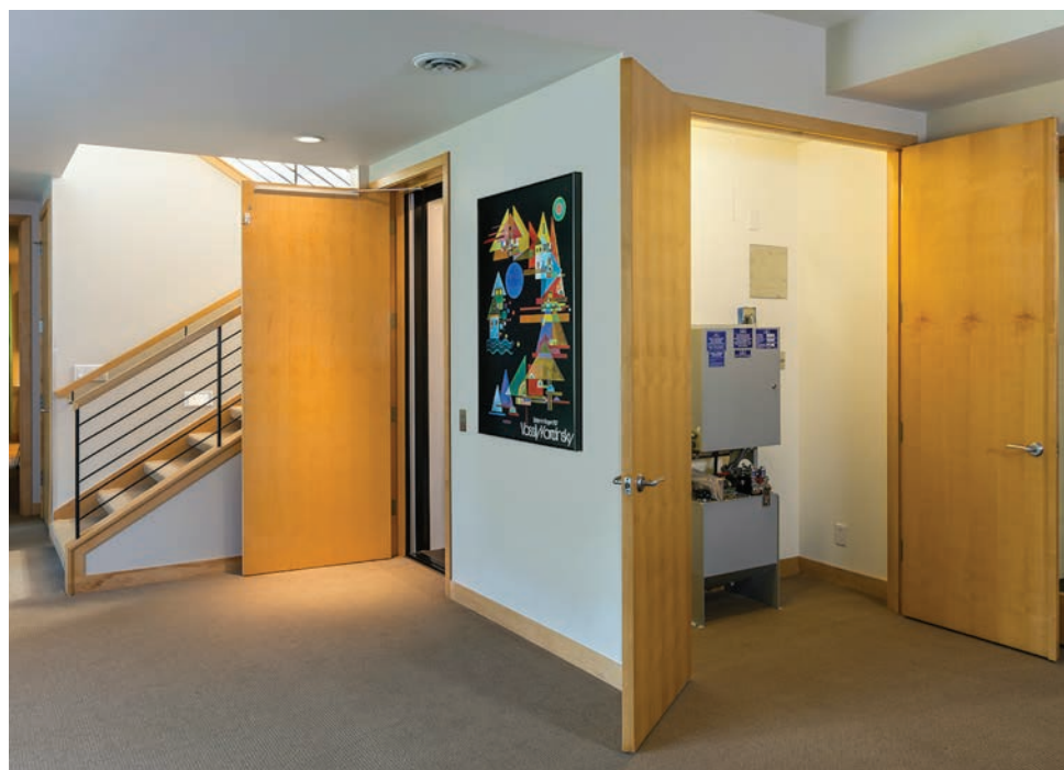
Installing a small elevator and widening doorways made this lower level more accessible. (Photo by Andrea Rugg Photography)
