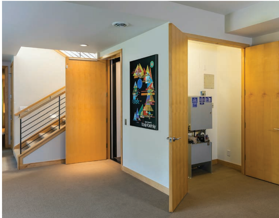
Installing a small elevator and widening doorways made this lower level more accessible. (Photo by Andrea Rugg Photography)
