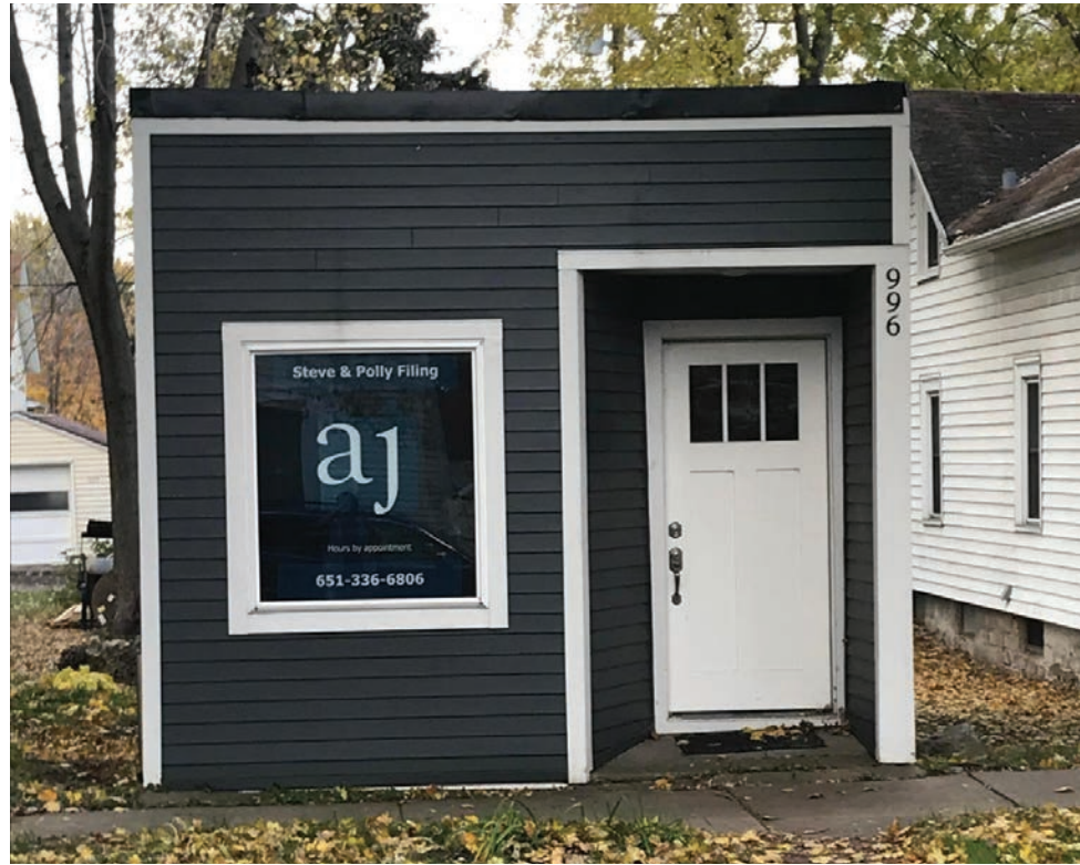
At 576 square feet, this office space at 996 Front Ave. is considered a small working space. "I just believe, whether it's for business or personal, you don't need as much space," said building owner Stephen Filing of Realty Group. (Photos submitted)
