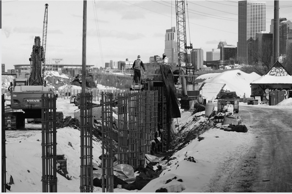
Construction of the corridor protection wall between Bryn Mawr Station and Glenwood Avenue in Minneapolis continues throughout the winter. Crews are seen preparing to pour concrete panels that form the wall. (Photo courtesy Met Transit)
