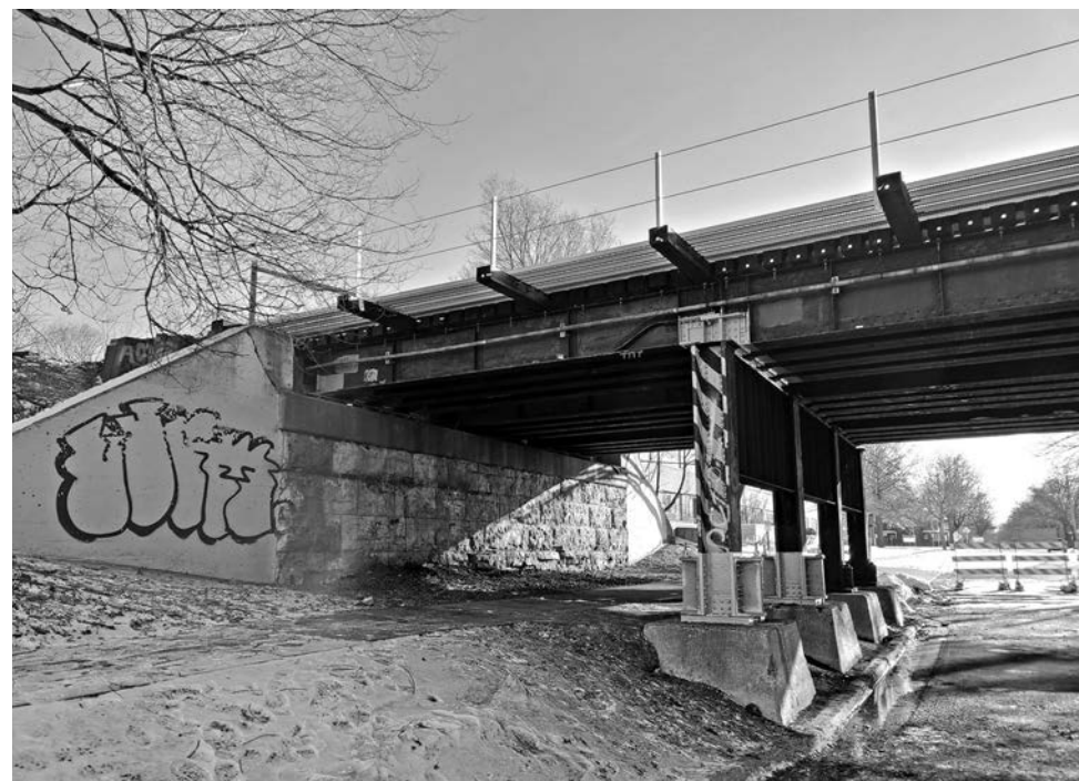
The newly completed repairs of the 31st Ave. railroad bridge include replacement of bearings, columns, column bases and related anchor bolts. (Photo submitted)
