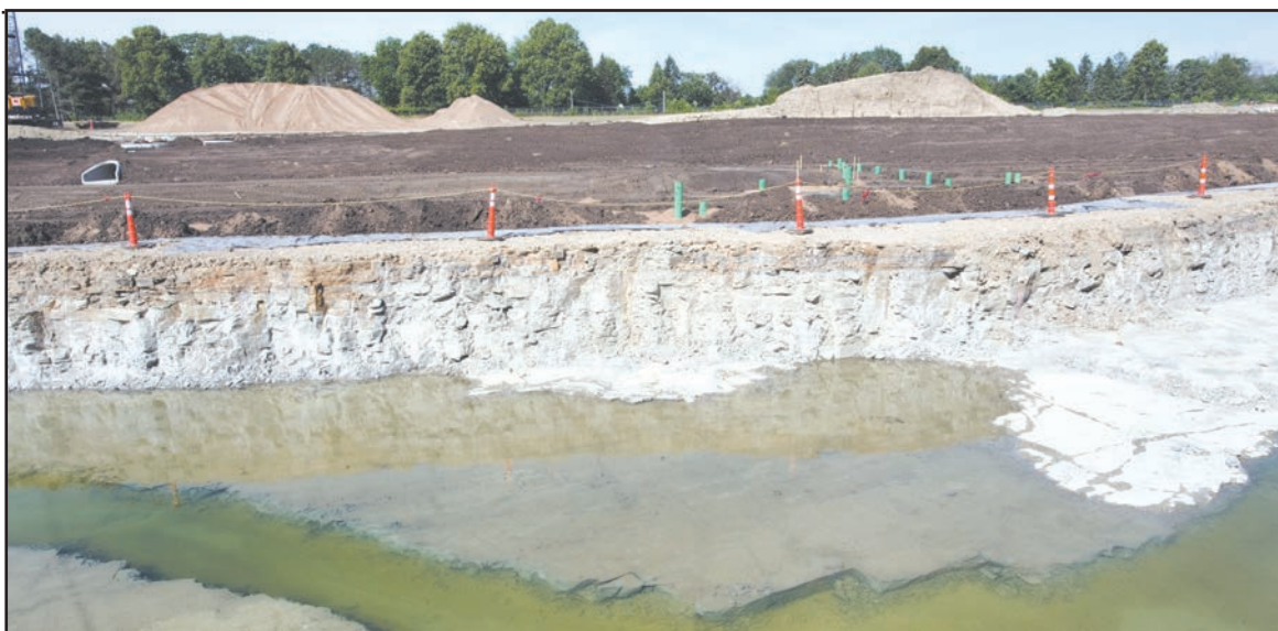
Green markers indicate where the manufactured wetland will be. Native plants growing in the wetland, along the water feature, and in surrounding rain gardens will help filter pollutants out of stormwater runoff. (Photo by Margie O'Loughlin)
