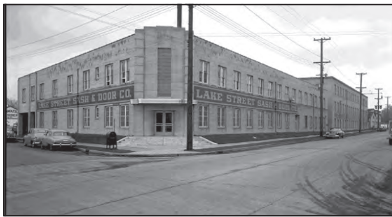
The Lake Street Sash and Door Company was the first, and soon a significant and longstanding millwork industry player along the Hiawatha transportation corridor. It was founded by Helmar Knudsen in 1916.
