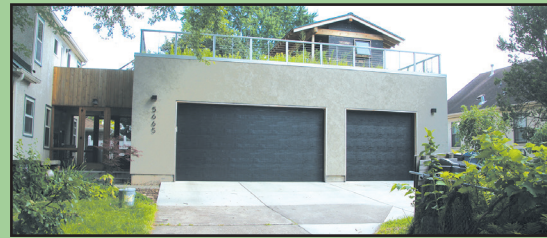
The green roof is part of an overall system for managing stormwater on site. The Musich family also overseeded the lawn with plants that help capture water and mow it at 4 inches. (Photos by Tesha M. Christensen)
