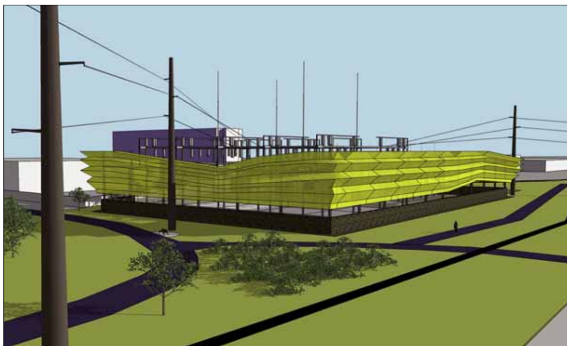
The graffiti-resistant walls of the new Hiawatha substation, located behind the Target building near the intersection of 28th and Hiawatha, will be illuminated yellow at night. The walls will be composed of extruded metal, a metal mesh surface that is semi-transparent. The metal will be given an anodized finish to color it and additional color will come from lighting. "This system is unique for this type of application," said Xcel Energy's Transmission Project Manager Joe Samuel. The substation will be complete in 2014. To follow the project, go to www.hiawathaproject.com .
