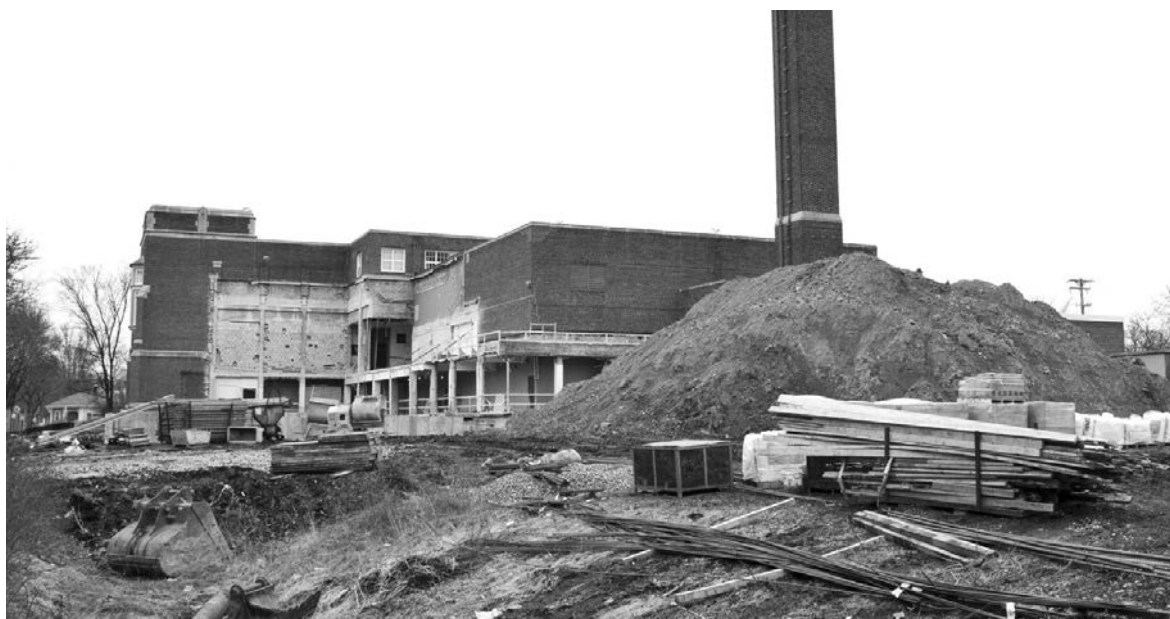
Construction of the new wing in full-swing. (Photo by Margie O'Loughlin)
